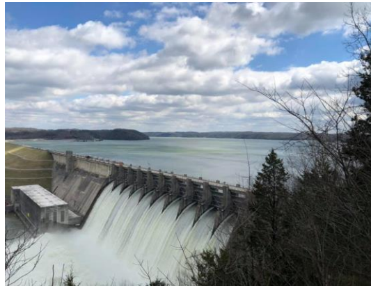
Wolf Creek Dam- Jamestown, KY
